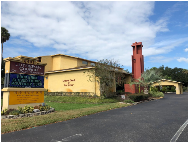
View when entering from Hills. Ave.
